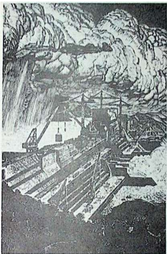
The construction site of a reservoir, by Chen Jinrong
