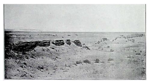
175- STRETCH OF ANCIENT BORDER-WALL, BUILT OK LAYERS OF REED FASCINES AND CLAY, EAST OF TOWER T. XIII., TUN-HUANG *LIMES*.
