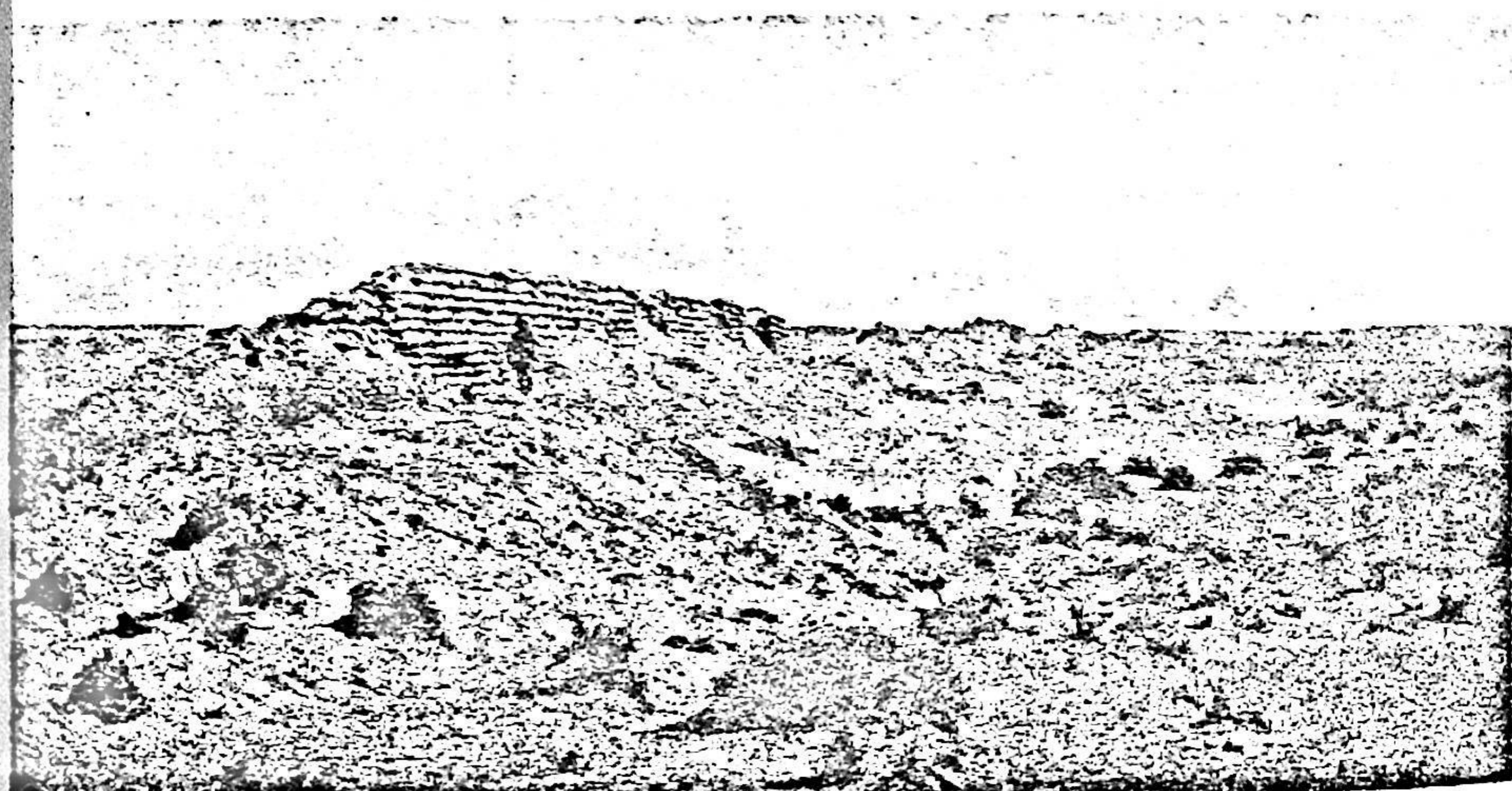
29 ANCIENT CHINESE BORDER WALL BUILT WITH LAYERS OF REED FASCINES, EAST OF WATCH-STATION 7.XIII., ON LIMES OF TUNHWANG
