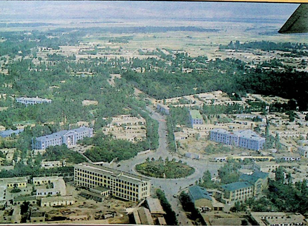
▼ 伊寧市俯瞰 Bird's-eye view of Yining City
